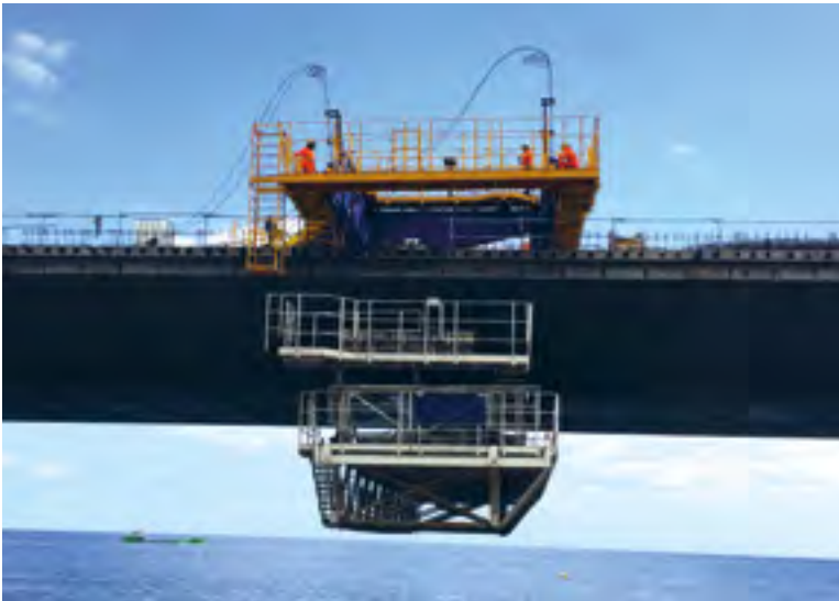
Saint-Denis (Reunion Island) — Grande Chaloupe viaduct work site.
