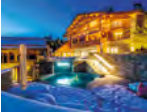
Megève — Eiffage Énergie Systèmes carried out the electrical engineering work for the La Cry hotel, which features 55 bedrooms and suites as well as a fine dining restaurant.
